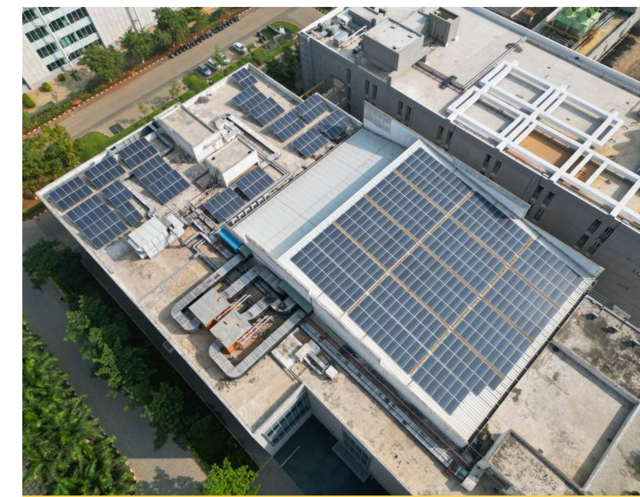
Solar Plant 180 KW
